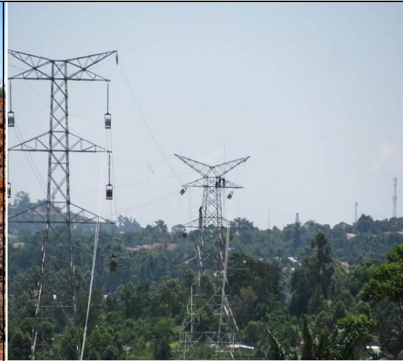
(b): Stringing Works near Kawanda Substation
