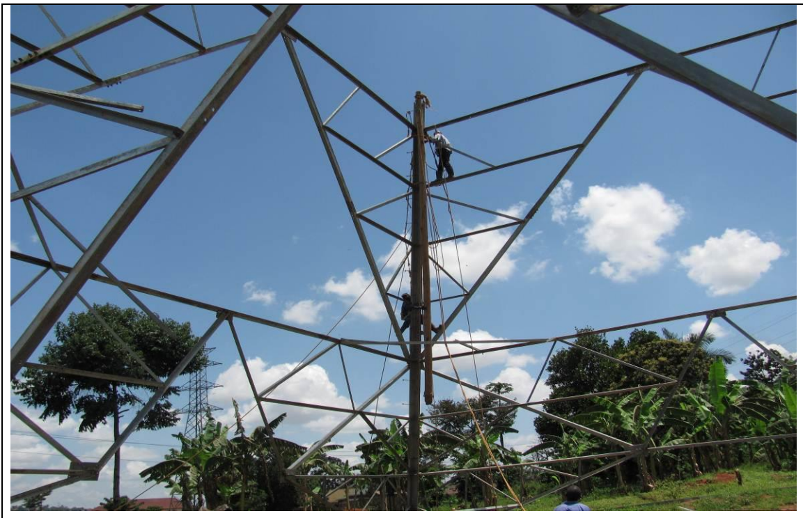
Employees erecting a tower without using the personal protection equipment , picture taken by OAG staff on 25th/10/2011
