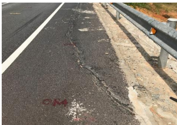
Picture 12: Crack in Asphalt due to settlement
