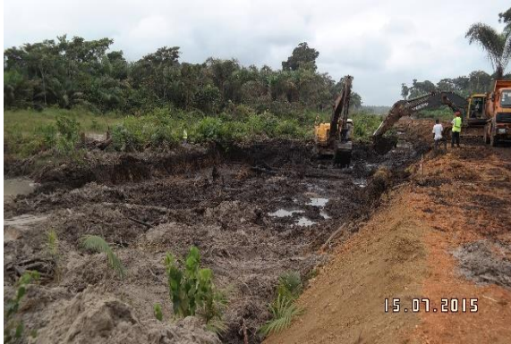
Picture 7: Filling of swampy section
