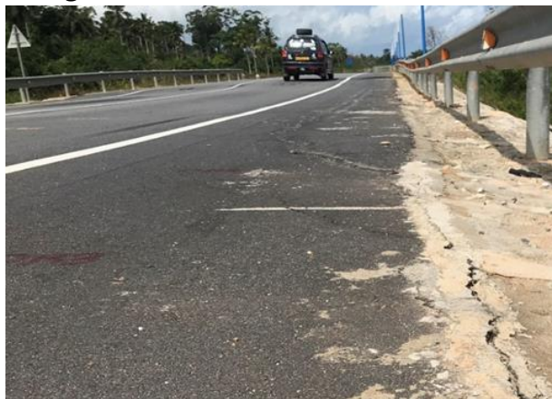
Picture 12: Crack in Asphalt due to settlement
