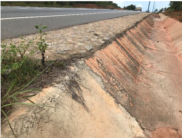
Picture 4: Stone pitching and trapezoidal drain
