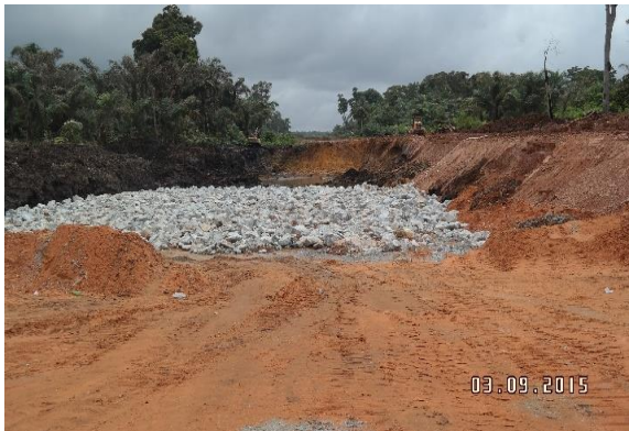
Picture 7: Filling of swampy section
