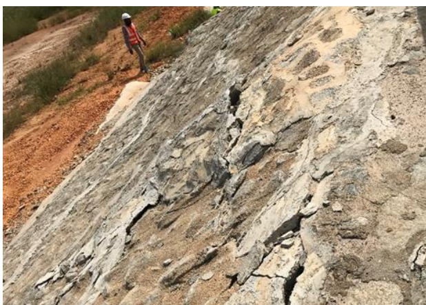
Picture 11: Crack in Embankment due to settlement
