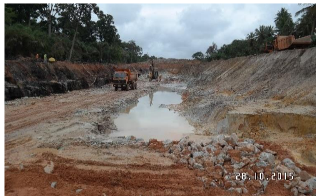
Picture 8: Filing and compaction of boulders
