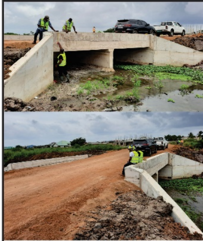
24. 280.00m x 4.00m x 2.00m reinforced concrete drain at Winneba Ntafakor. (Redesigned to 10.5m x 8.5m x 1.5m box culvert-45% completed)
