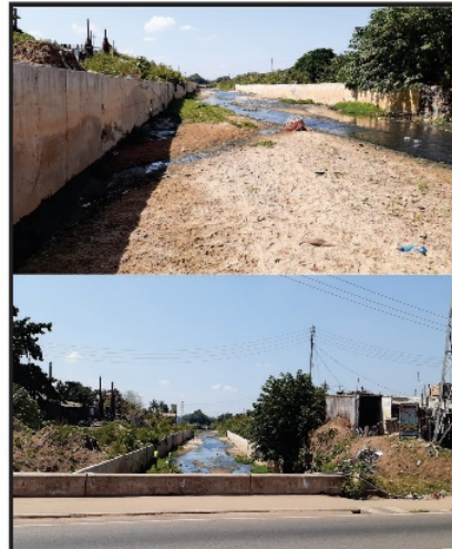
19. 305.00m x 16.00m x 2.50m reinenforced concrete drain at Kumasi Aboabo. -23% completed
