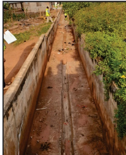
17. 411m x 2.7m x 1.60m reinforced concrete drain at Ejura- 33%
