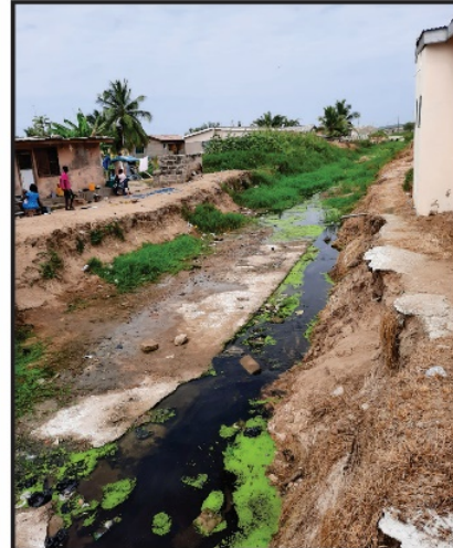
23 280.00m x 3.00m x 1.50m reinforced concrete drain at Winneba Salt Pan (project at stand still - 0.1% completed)
