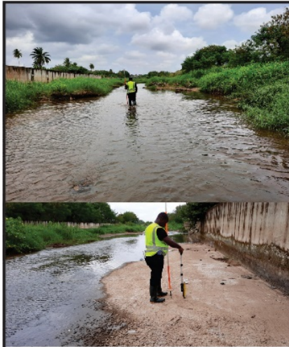
22. 2200m x 25.0m x 2.5m reinforced concrete drain at Akora (Agona Swedru) -40% completed
