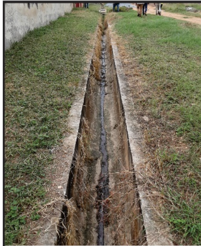
11. 420m x 0.60m x 0.60m concrete U-drain at North Legon -100% completed
