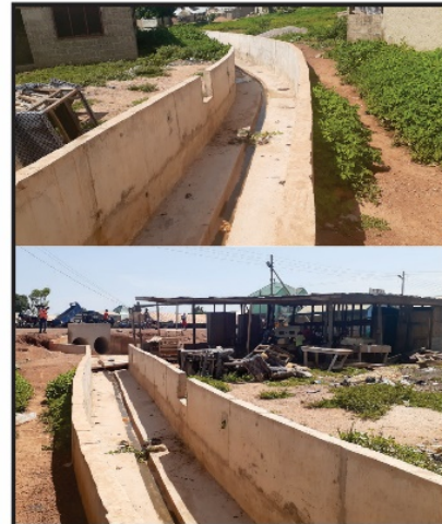
27. 60.00m x 3.00m x 1.50m reinforced concrete drain at Zebilla. (Redesigned to 120m x 2m x 1.5m reinforced concrete drain-100% completed)
