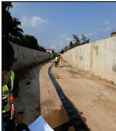
2. 600m x 3.7m x 2.50m reinforced concrete covered drain at South Nima. (Redesigned to 250m x 8m x 2.5m reinforced concrete drain & culvert and relocated to Haatso -55% completed)
