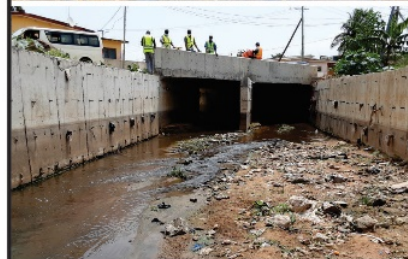
9. 120.0m x 7.00m x 2.50m reinforced concrete open drain at Mallam. (Redesigned to 2no., 23m x4m x 2.5m and 16m x 9m 2.5m box culverts -52% completed)
