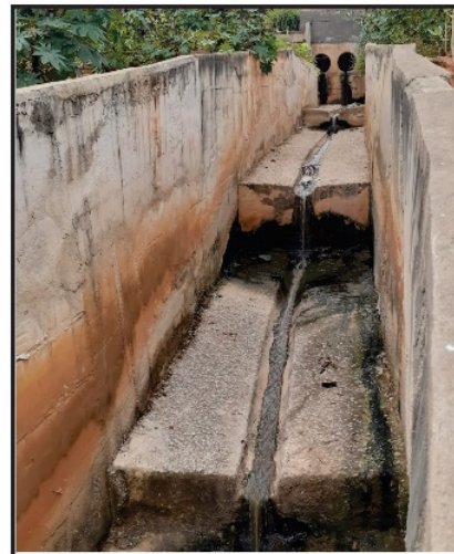
21 42.00m x 3.30m x 1.80m and 89.00m x 2.00m x 1.60m reinforced concrete open drain at Tapa (lot 1) -100% completed
