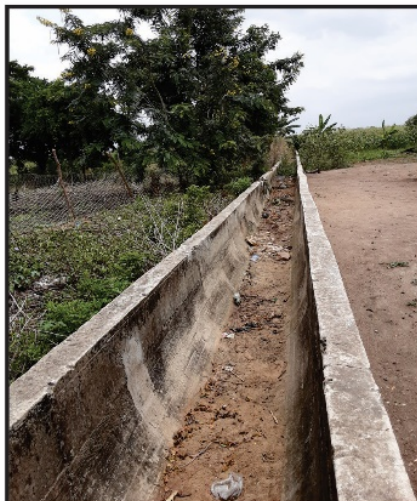
14. 130.0m x 0.90m x 0.90m concrete U-drain at Osuwem- 100% completed
