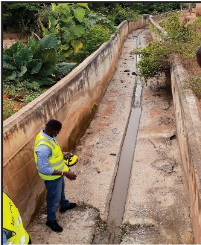
16 Pipe drain size 1.5m (diameter) x 131m (length) at Tepa (lot 2) (Redesigned to 150m x 2.0m x 1.5m rein. conc. drain-22% completed)
