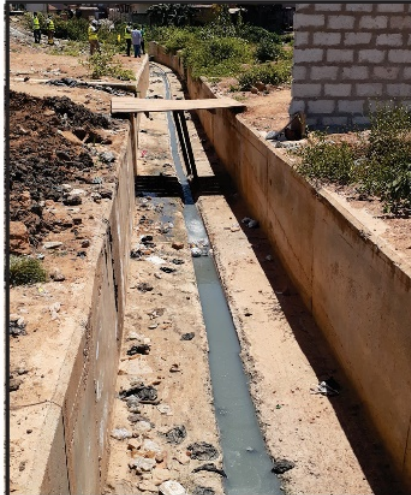
18 165m x 3.5m x 2.00m rein.concrete drain at Kumasi Amakom E.P Church. (Redesigned to 350m x 2m x 2m rein.concrete drain-100% completed)
