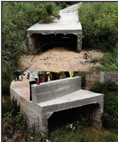
10. 125.00m x 2.50m x .50m concrete covered drains and 900.00m x 0.75m x 0.750m concrete U-drain at New Ningo -25% completed
