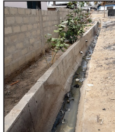
3. 180.0m x 2.50m x 1.50m reinforced concrete open drain at Sukura. (Redesigned to 370m x 0.9m x 0.9 concrete U-drain - 100% completed)
