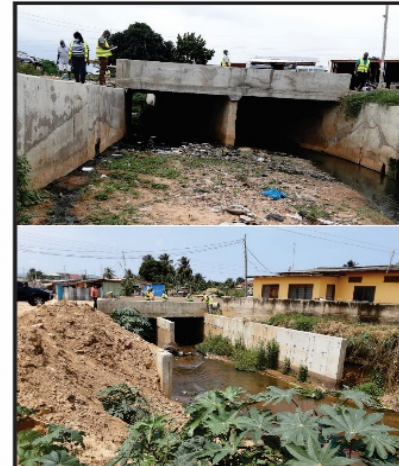
1. 165m x 3.50 x 2.00m reinforced concrete covered drain at Santa Maria. (Redesigned to 2 no., 20m x 5m x 2.5m and 16m x 9m x 2.5m box culverts- 100% completed)
