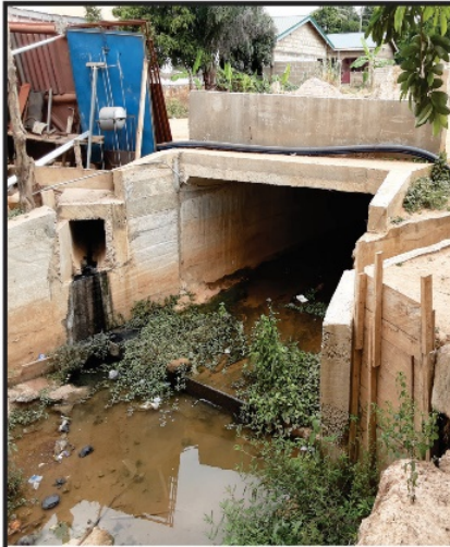
4. 15.00m x 3.50mm x 1.50mm reinforced concrete open drain at Ashiyic. (Redesigned to 16m x 4m x 2m box culvert- 100% completed)
