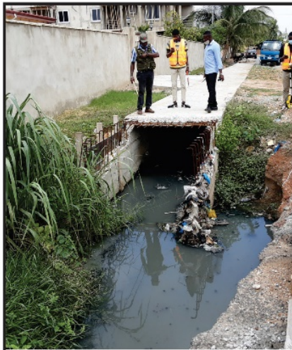
6. 21.50m x 3.6m x 1.70m rectangular concrete drain at Kordjor. -25% completed
