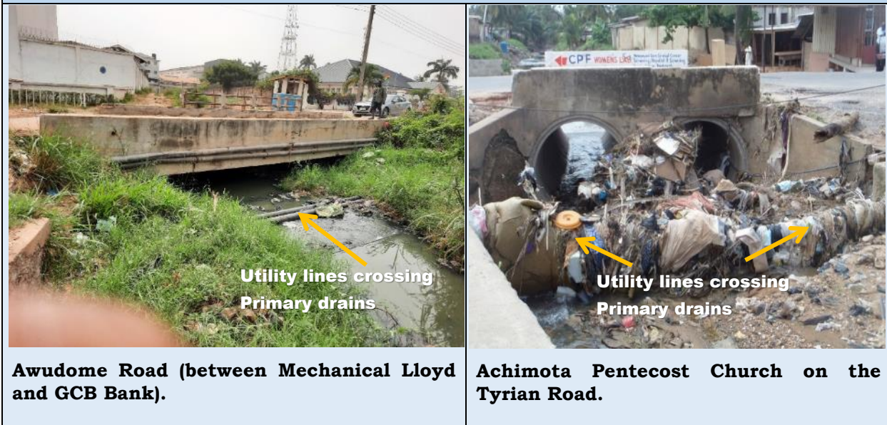
Picture 6: Examples of utility lines crossing drainage facilities.
