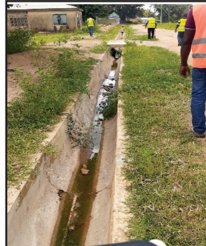
25. 230.0m x 3.00m x 1.50m reinforced concrete drain at Bolgatanga, Kumbosco. (Redesigned to 1000m x 0.6m x 0.6m U drain-61% completed)
