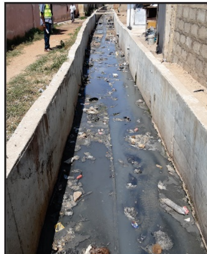
7. 250.0m x 3.50m x 1.50m reinforced concrete open drain at Abeka Lapaz (2018). (Redesigned to 350m x 2.0m x 1.3m rein.conc. drain -100% completed)
