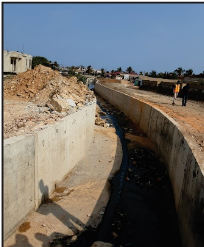
12. 250.0m x 3.50m x 1.50m reinforced concrete drain at Nungua. (Redesigned to 250m x 3.0m x 1.8m rein. conc. drain-95% completed)
