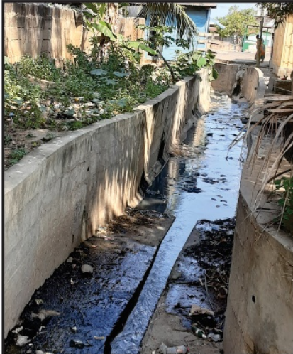
8. 90m x 2.50m x 1.00m rectangular plain concrete drain at Abeka Lapaz (2017). -100% completed
