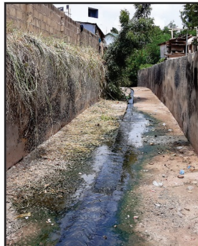
5. 21.50m x 3.6m x 1.70m rectangular reinforced concrete drain at East Legon, – 100% completed
