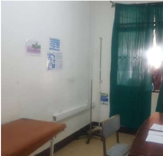
Photo 3.9(a): Patient's resuscitation room with no emergency equipment for treatment
