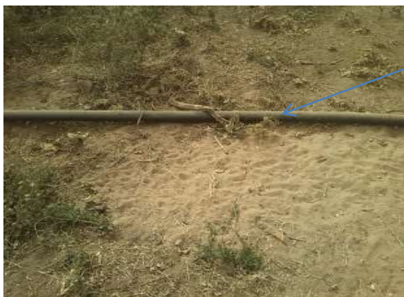
Photo 3.4: Pipe laid on the ground instead of being one meter below the ground
