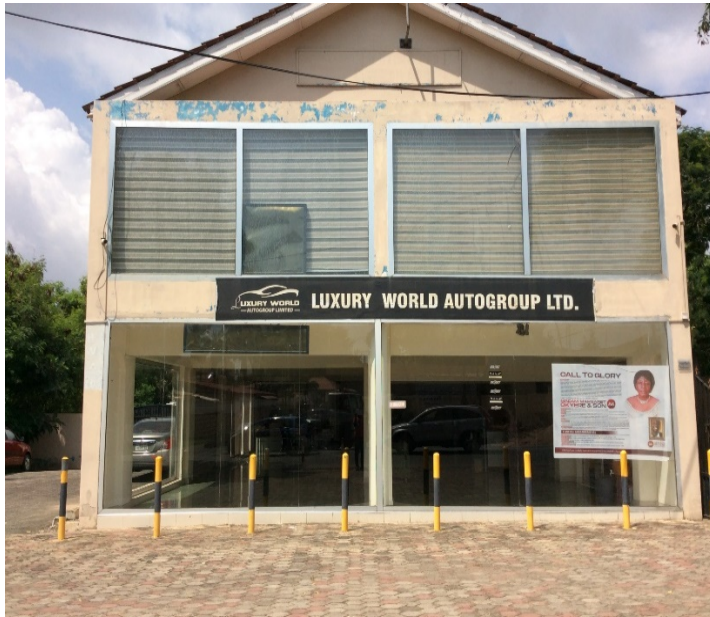
Picture 9: Office of LWAGL at East Legon in Accra used as SGAGL Workshop
